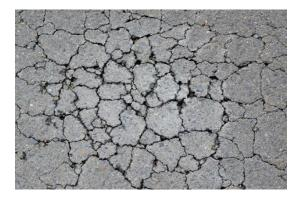
crack filler is that it could potentially stick to the tires of the car and cause worse damage. The proper repair for these areas should be saw cut out and replaced with new asphalt.
